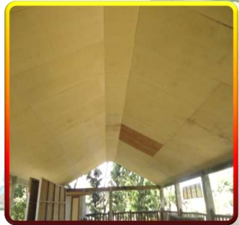
Completion of Ceiling at the Alumni Building
