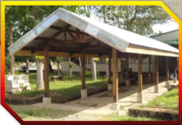
Covered Walk at CE Building
